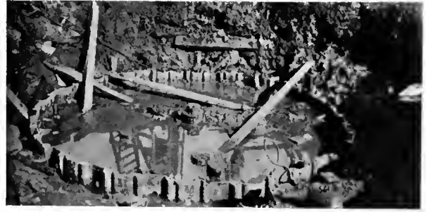
CLOSE-UP OF CYLINDER AFTER DRIVING
